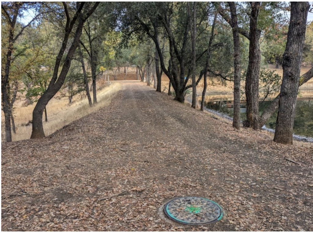
Bass Pond's dam crest showing trees growing in it and the community sewer line access port in the foreground.
