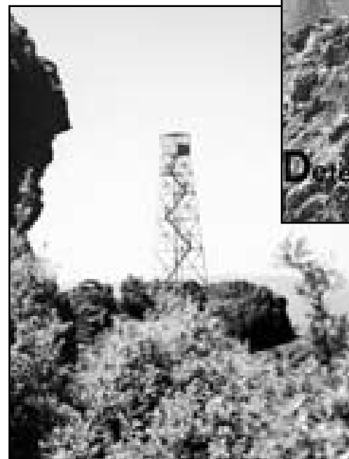
Above: Looking up Yosemite Valley, the Stanislaus National Forest Lookout on Trumbull Peak was built by the CCC from 1934-35. The site — awaiting restoration — includes a 41' steel tower with 7' x 7' metal cab plus a 19' x 30' C-2 quarters built partly on stilts because of the steep terrain. The bedroom resembles a lookout with windows on three sides.
