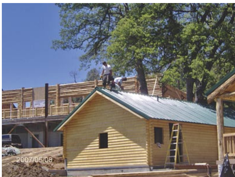
Dalrymple Construction puts the roof on a bathhouse.
