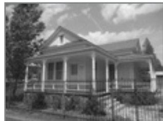
Cobden House 2016 after preservation.
