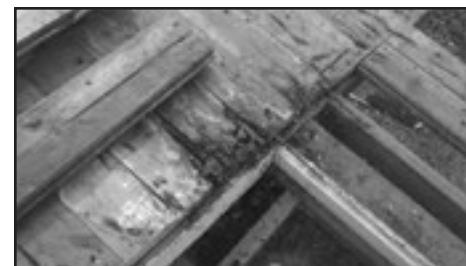
This is an example of the repairs that need to be completed to the restroom on #13.
