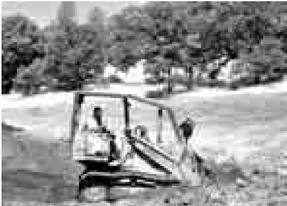
Down to Earth employee start digging the camp pool.
