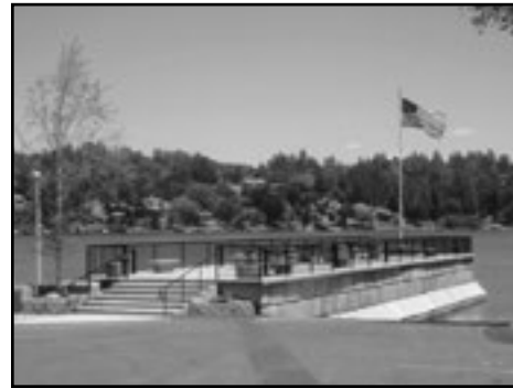
The new and improved Marina Jetty.
