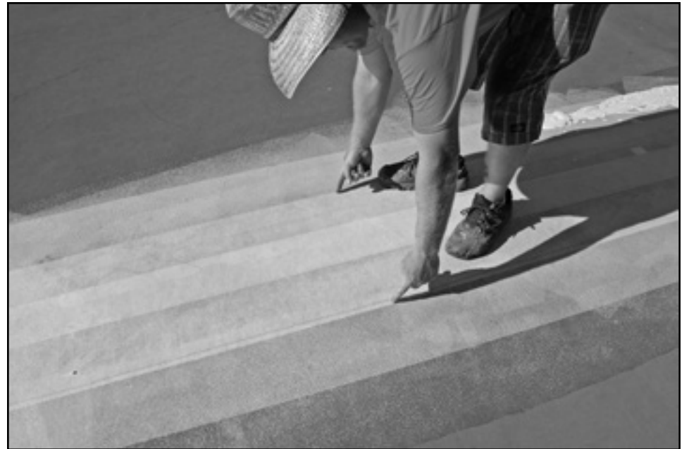
The patch material applied over the cracks, much like a band-aid.
