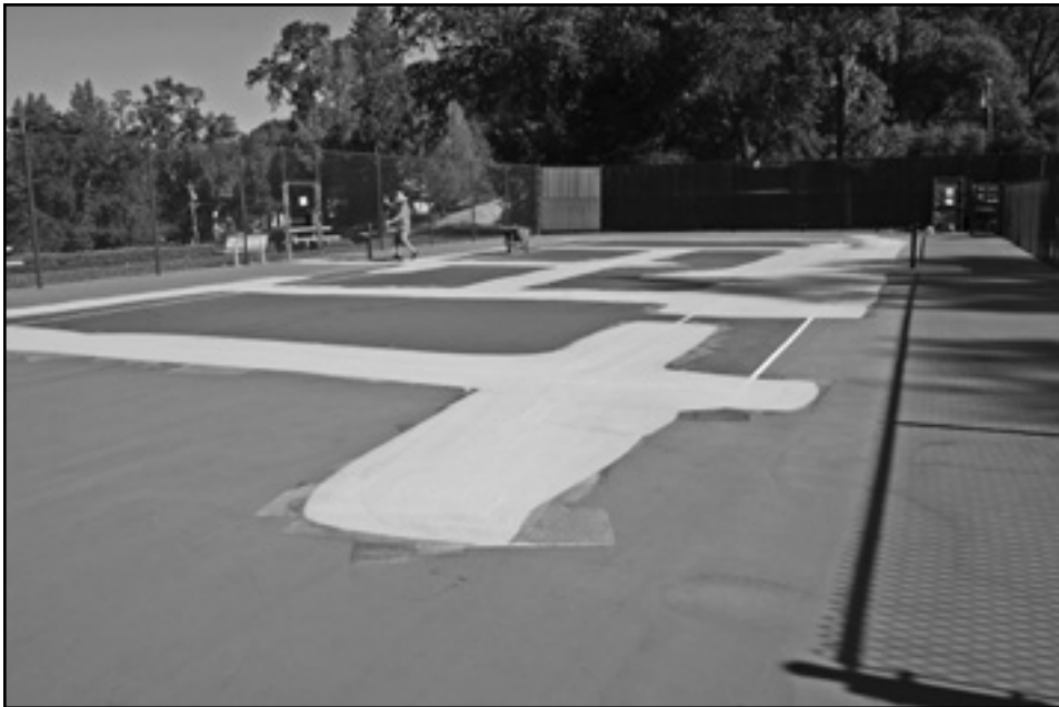
The patches applied to the cracks on the courts.
