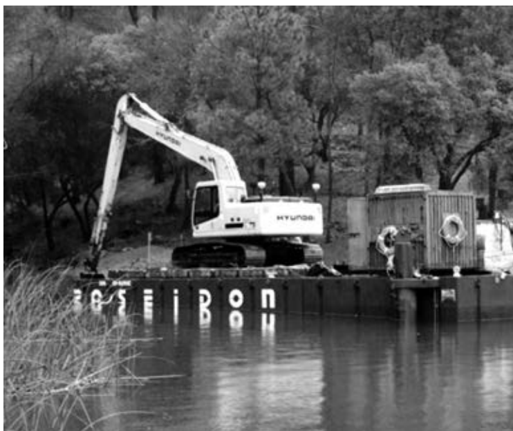
Dredger at work in Fisherman's Cove
