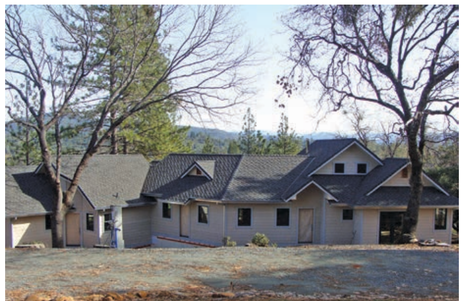
Currently under Construction Custom Designed on 8 acres in Groveland
